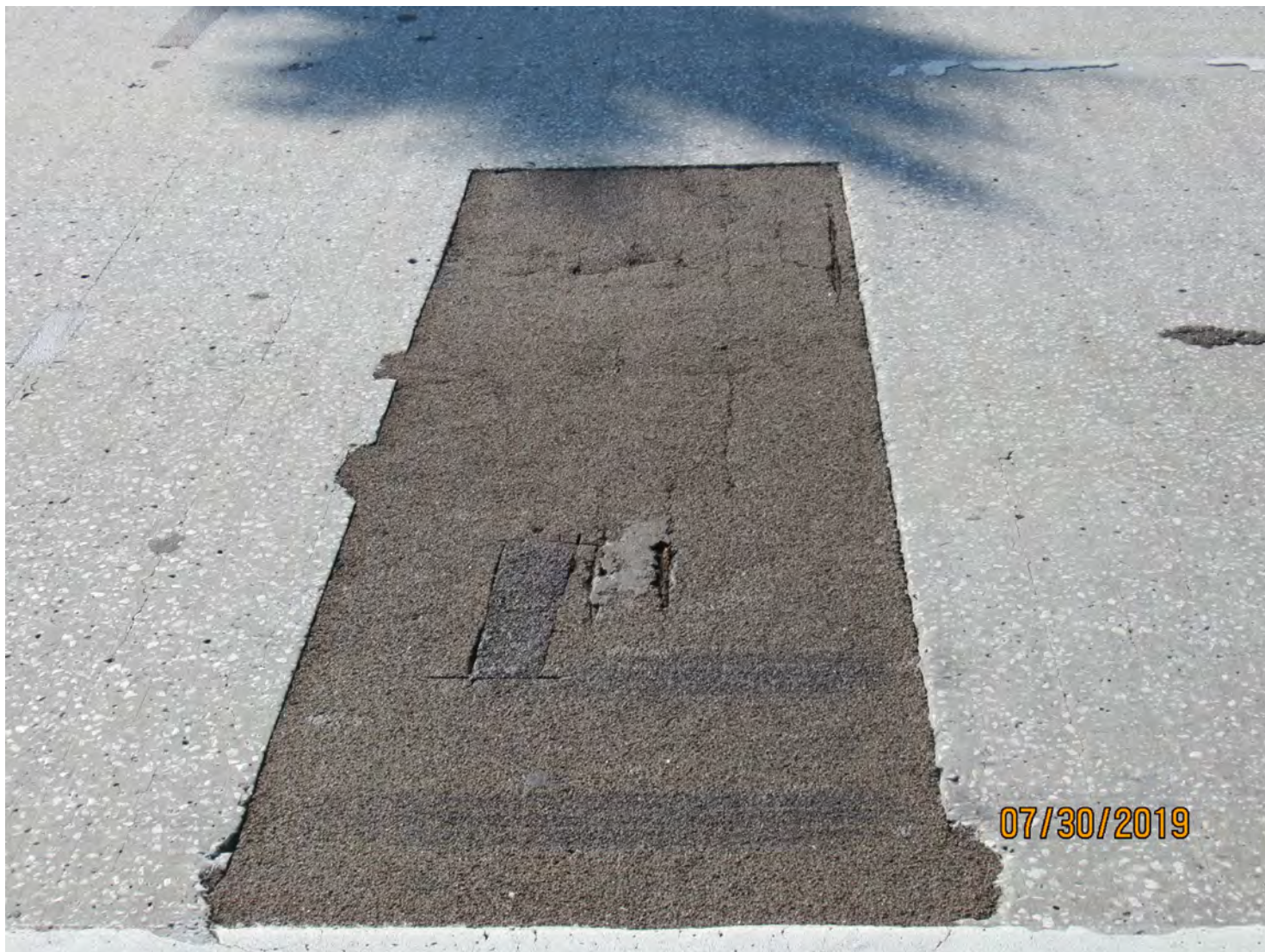
Photo 1: Element 12 Re Concrete Deck
