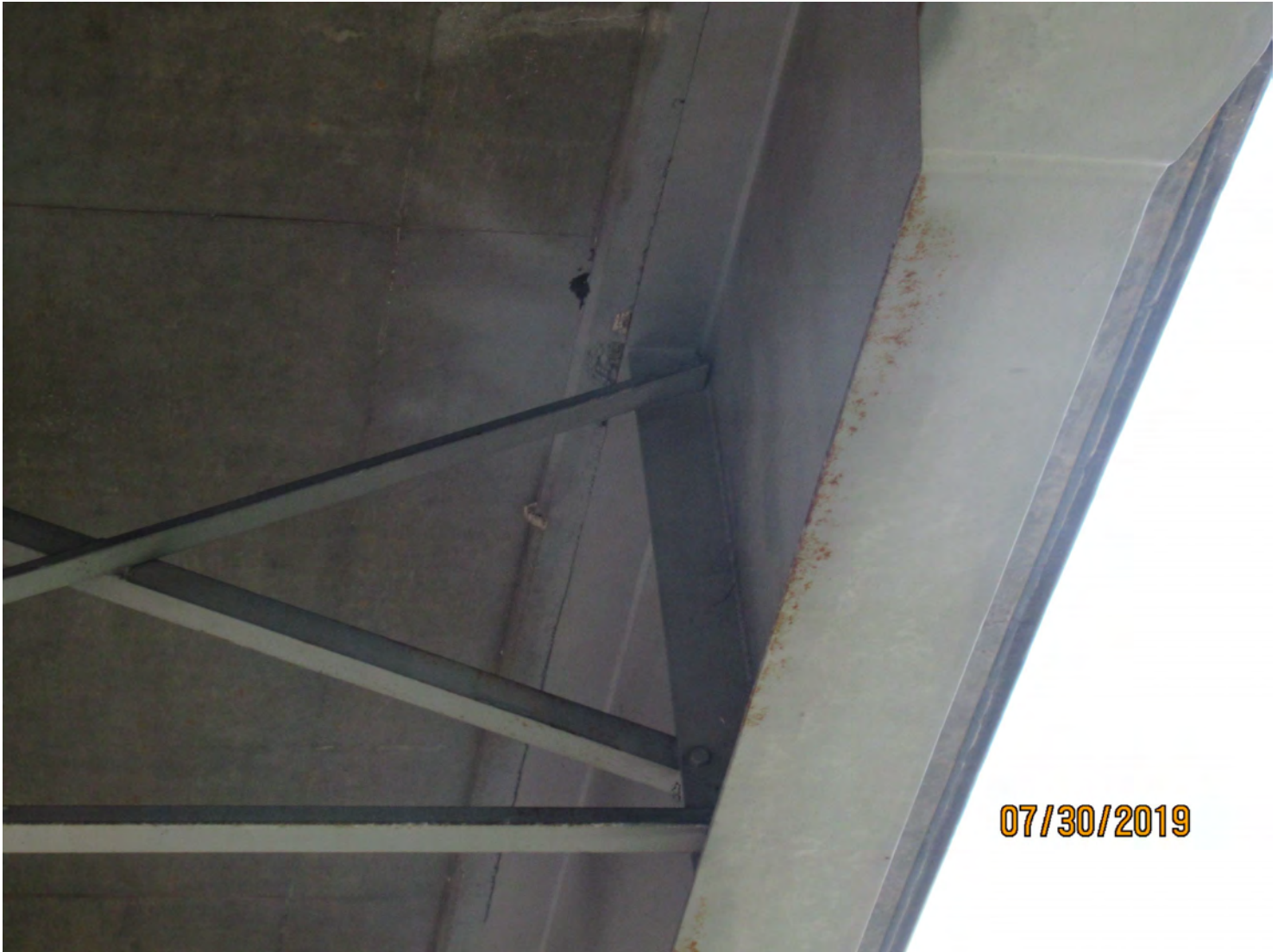
Photo 7: Element 107 Steel Opn Girder/Beam
