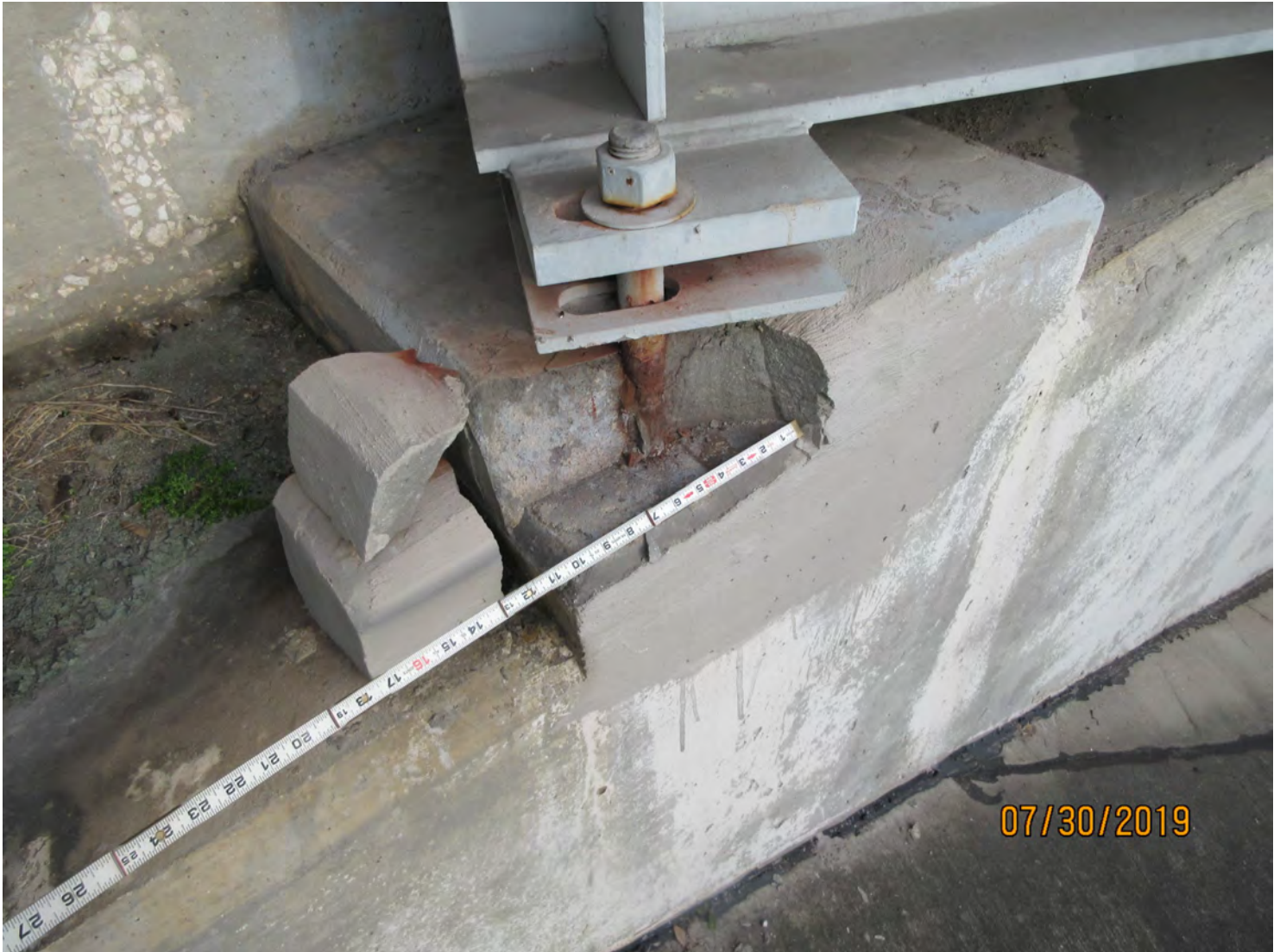
Photo 7: Element 215 Re Conc Abutment
