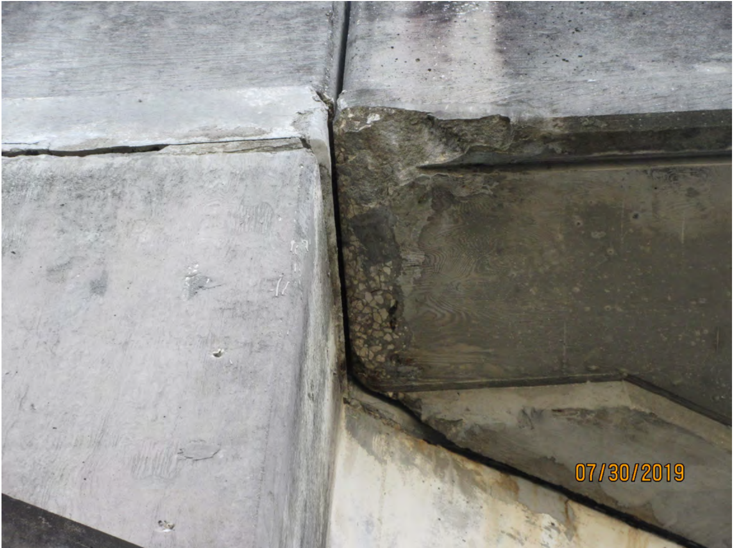
Photo 2: Element 12 Re Concrete Deck
