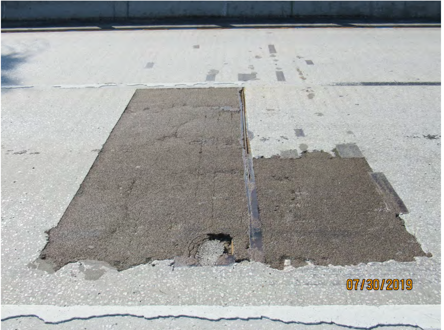
Photo 2: Element 12 Re Concrete Deck
