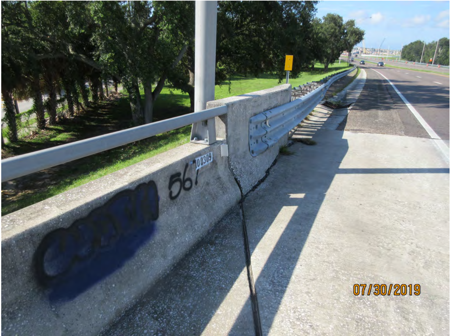
Photo 8: Element 333 Other Bridge Railing
