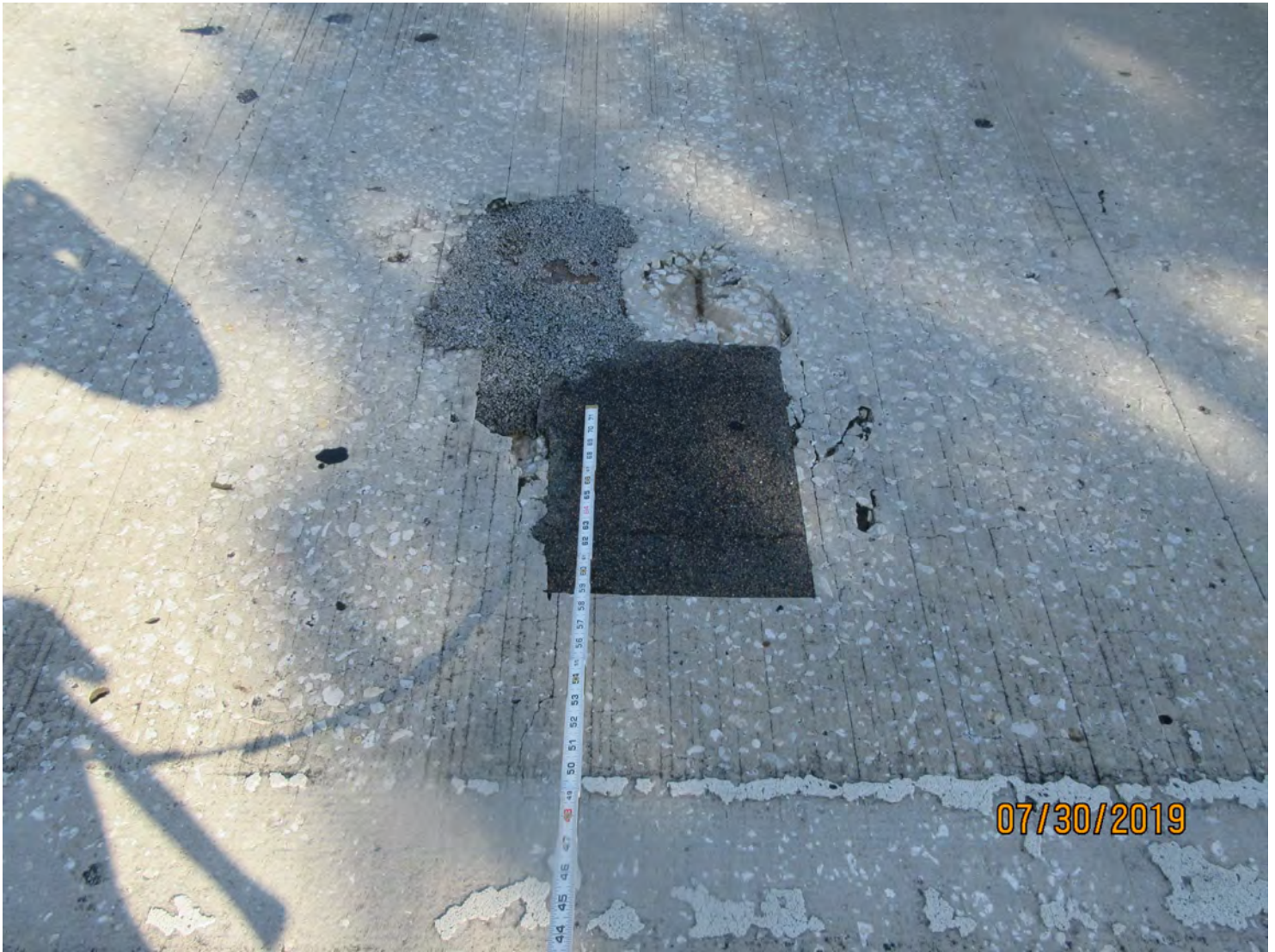
Photo 1: Element 12 Re Concrete Deck
