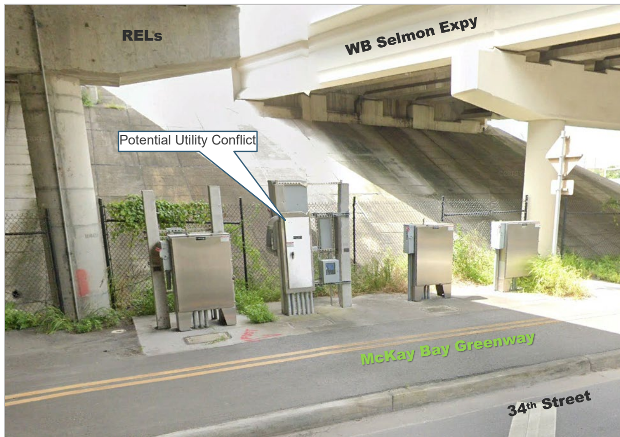
Figure 8: Existing utility cabinets under 34th Street bridge (Source: Google Earth)
