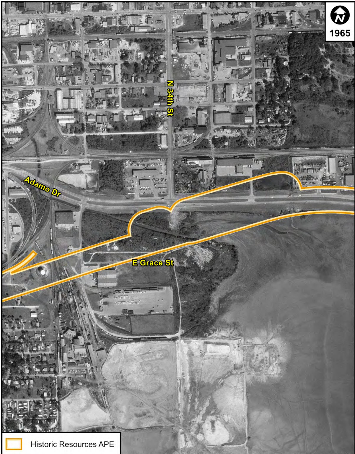
Figure 4: A 1965 historic aerial photograph of the project area surrounding the proposed Egress Ramp by the I-4 Connector (Ramp 2)
