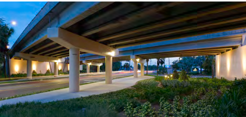
Selmon Expressway overpass at Swann Avenue
